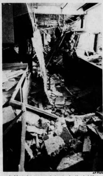
An Atlanta day care center lies in ruins after Monday's blast.
