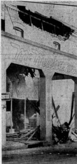
QUAKE DAMAGED THIS BUILDING ... near epicenter in Calexico
